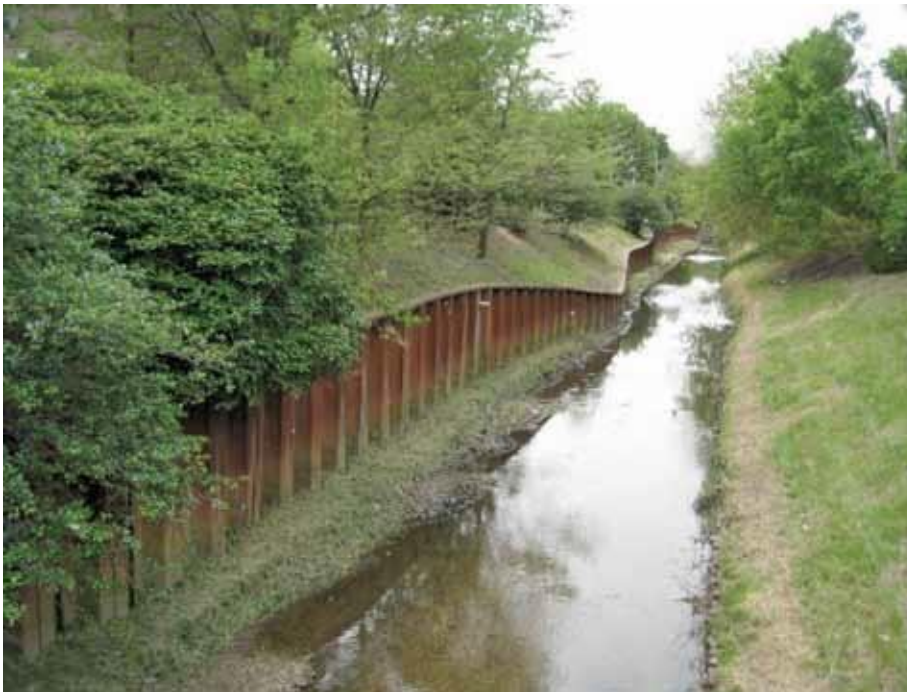
Photograph 3Q-1. A well maintained section of Weller creek where bank stabilization has been installed. Creek and drainage maintenance is important to keep trees and branches from blocking drainage, stabilizing creek banks and protecting property flooding and erosion, and to eliminate breeding locations for pests.
